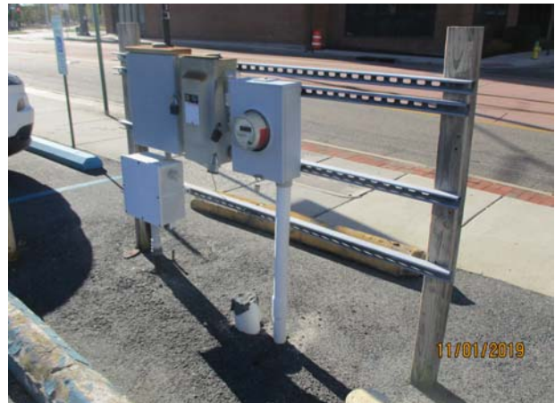
Photograph 8. Electrical panel assumed to be associated with on-site lighting.
