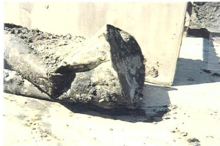
UST 1 was crushed prior to removal. Bottom View of UST 1.
