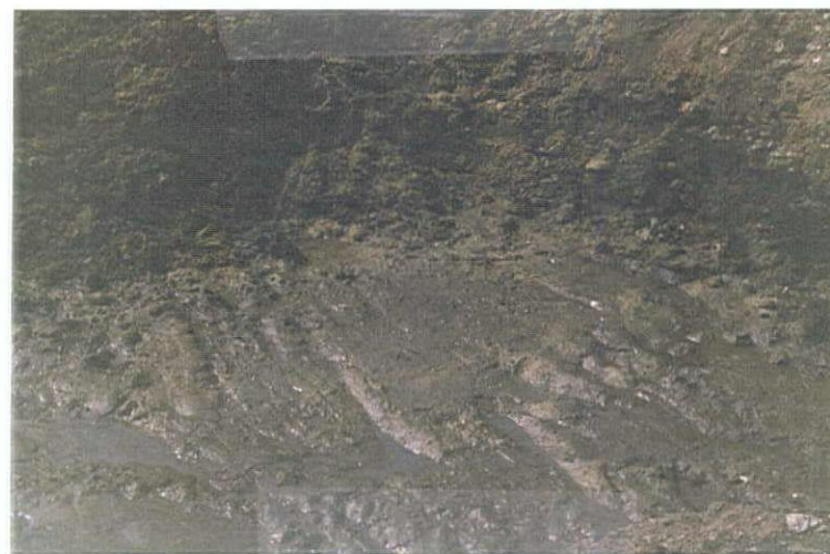
Excavation after the removal of petroleum impacted groundwater.
