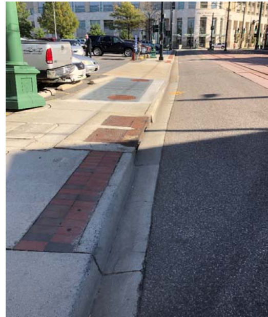
Photograph 20. Stormwater inlet on E. Plume St.
