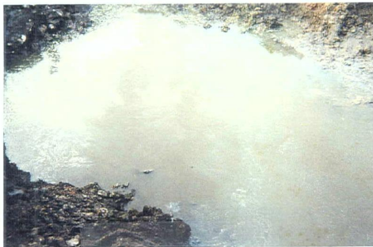
Free Floating product on the surface of the groundwater recharge in the excavation.
